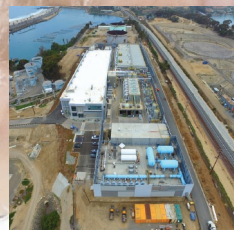
Claude "Bud" Lewis Desalination Plant in Carlsbad
