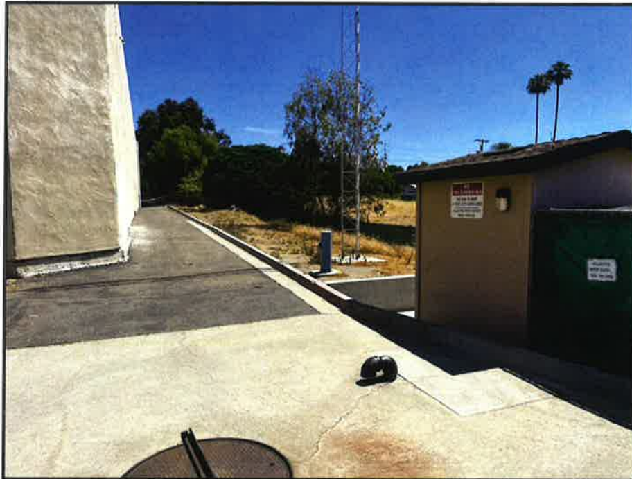
View to the northeast from the sewer lift station toward the location of the proposed easement.
