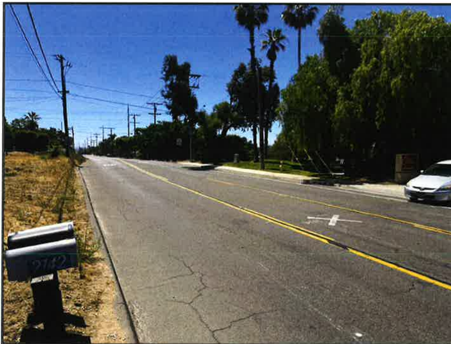
View to the southeast along Montiel Road with the subject larger parcel visible at the right.
