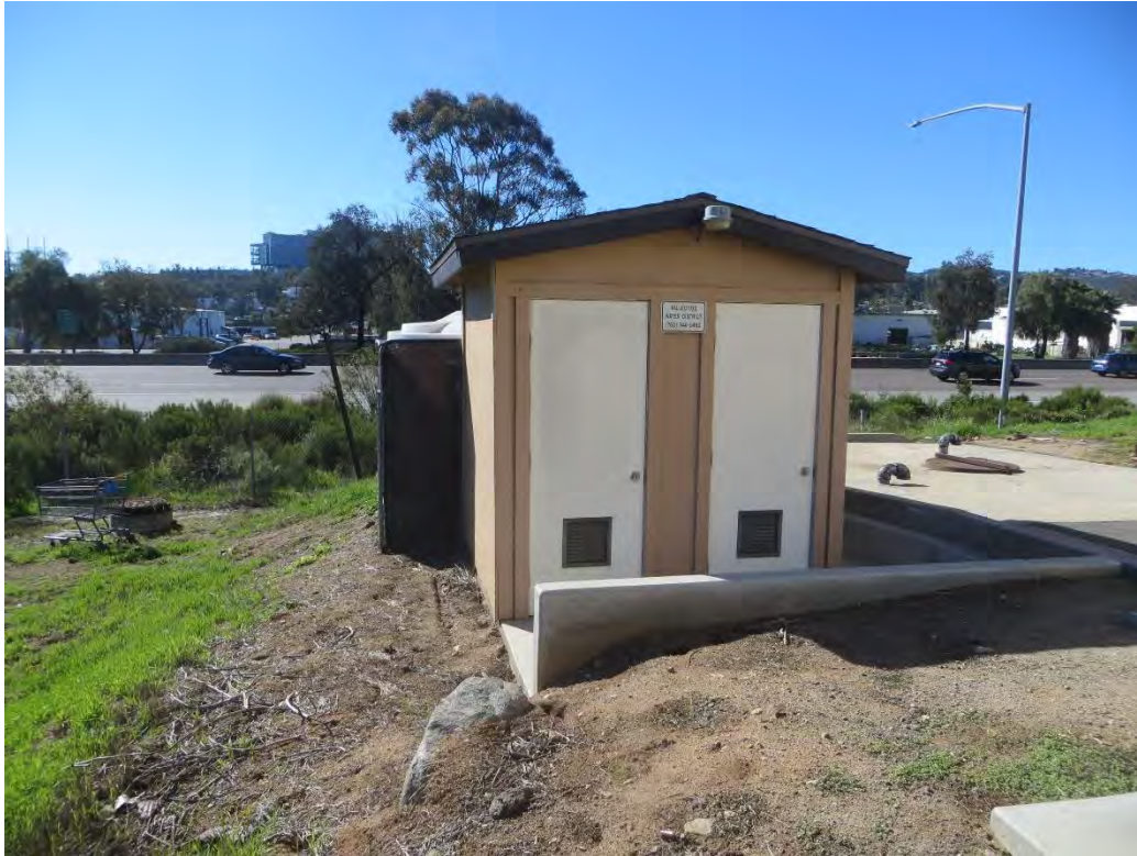
Photograph 9: Facing southwest at the Montiel Lift Station.
