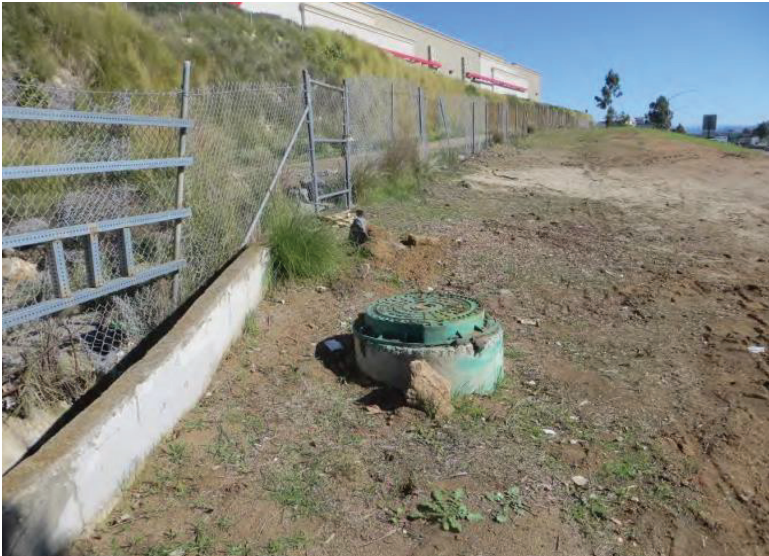
Photograph 1: Standing at the western end of the project, facing east at one of two manholes located along the western terminus.
