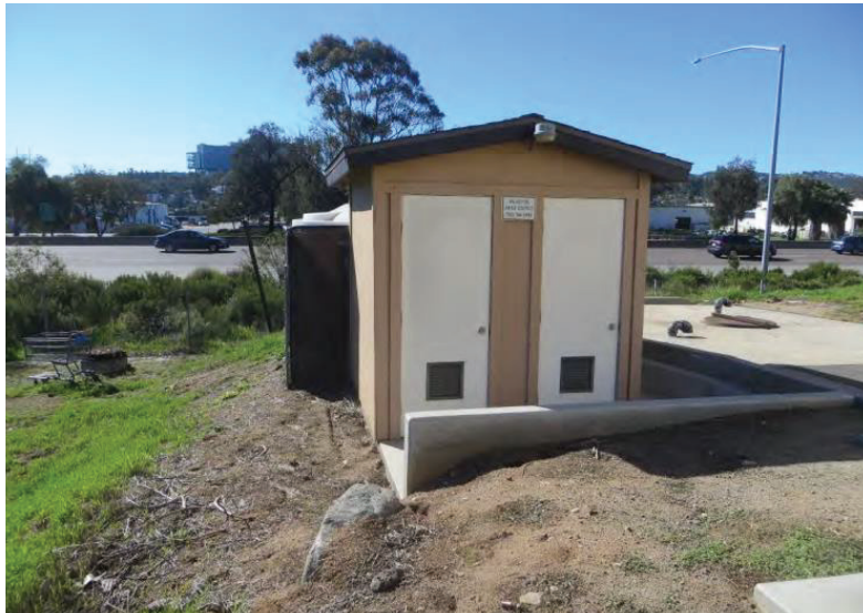
Photograph 7: Facing southwest at the Montiel Lift Station.
