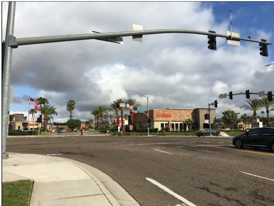
Figure 8. Nordahl Road at intersection with Montiel Road (view northwest). May 13, 2020.
