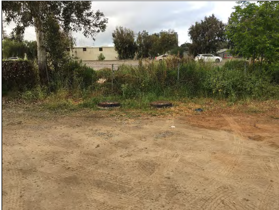
Figure 3. Manholes at southern end of Kaylyn Way (view south). May 13, 2020.
