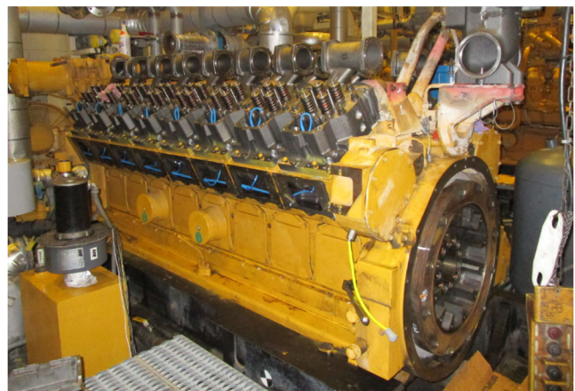
Overhaul on a 1,000 horsepower engine
