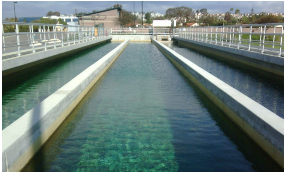
Carlsbad Water Recycling Facility
