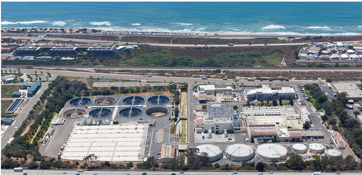
Encina Water Pollution Control Facility
