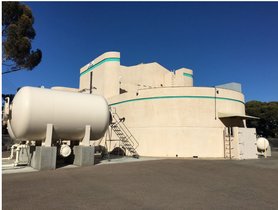
Buena Vista Pump Station
