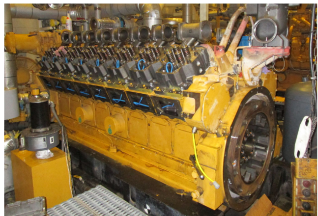
Overhaul on a 1,000 horsepower engine
