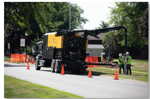
Figure 2: Typical Potholing Setup
