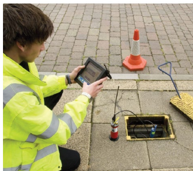
Figure 3: Leak Detection Noise Loggers
