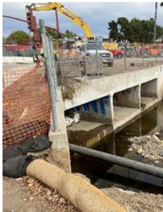
Existing Triple Box Concrete Culvert in San Marcos Blvd
