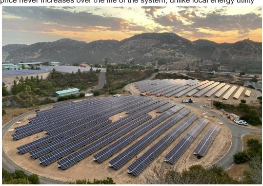
The system at LS1 will offset approximately 90% of the energy demand at that location. The larger system at Twin Oaks Reservoirs will offset approximately 57% of the remainder of our system electricity demand.
