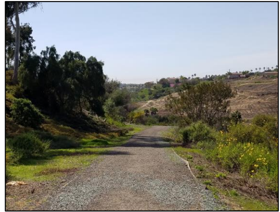
The Land Outfall is a critical component of the District's infrastructure. The alignment includes narrow easements along environmentally sensitive corridors and major streets.
