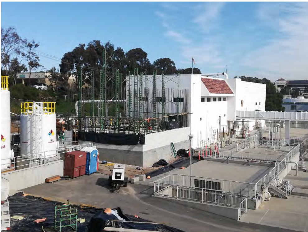
Expansion of the Headworks Building
