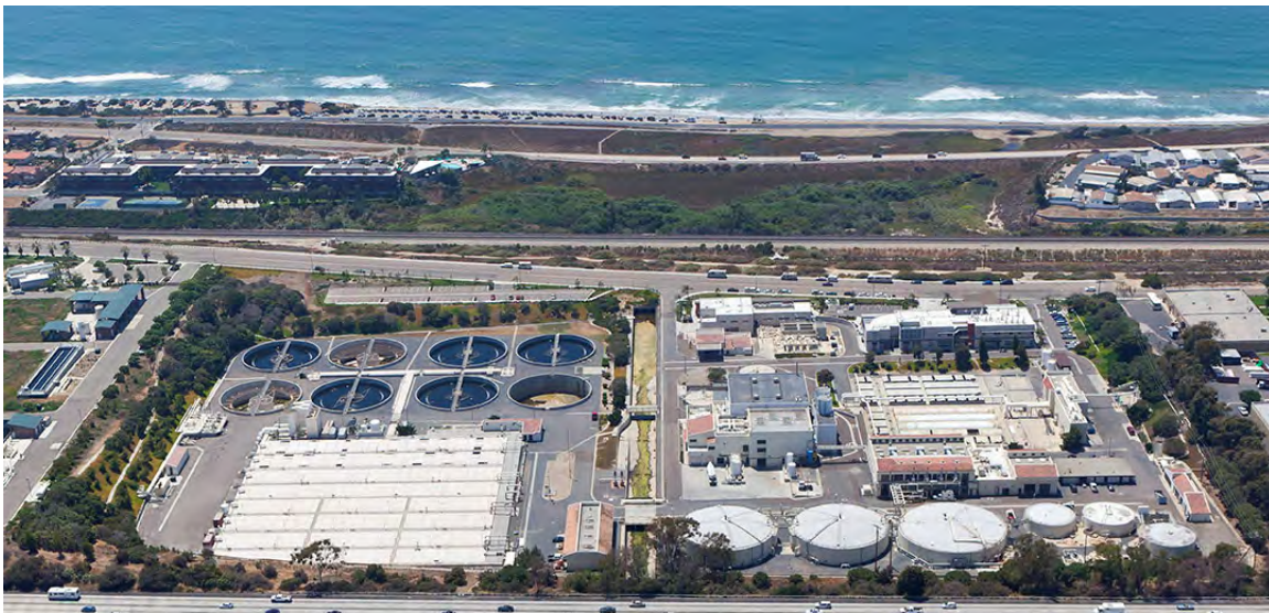
Encina Water Pollution Control Facility
