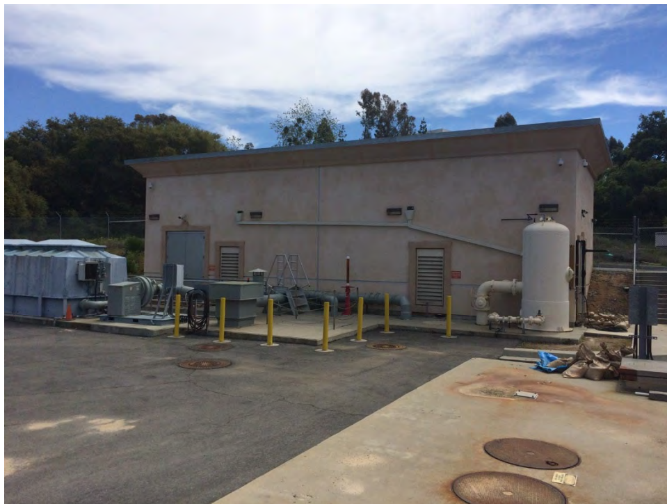
Buena Creek Pump Station
