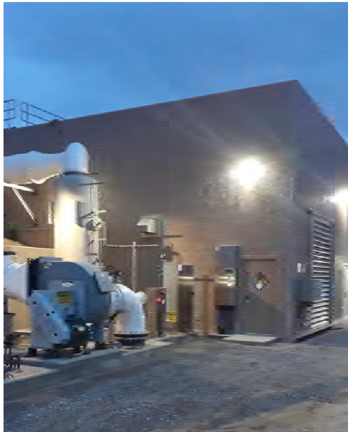
Newly Constructed Agua Hedionda Pump Station
