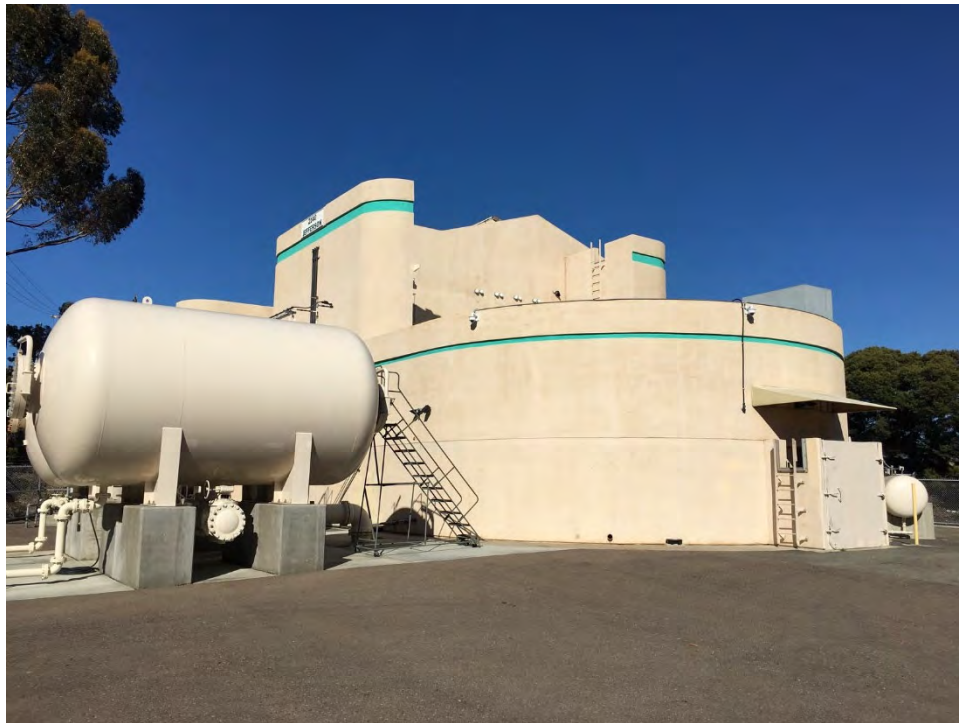
Buena Vista Pump Station
