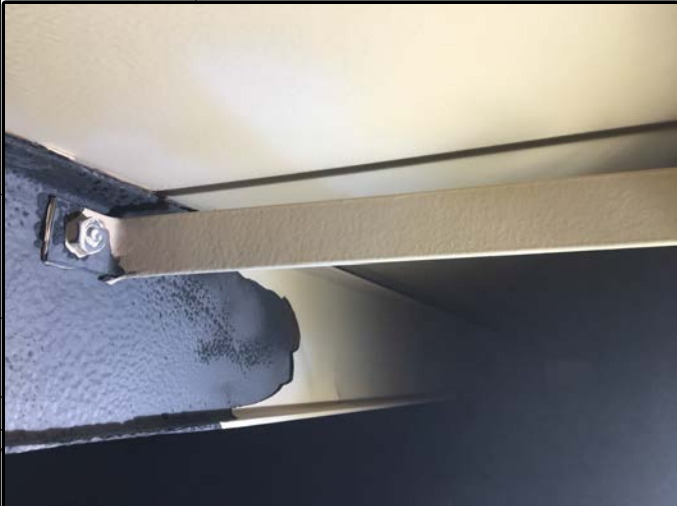
BLAST INSPECTION - INTACT RAFTER
