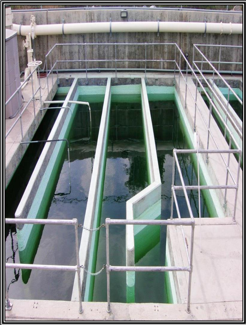
Chlorine Contact Tank at Meadowlark Wastewater Reclamation Facility
