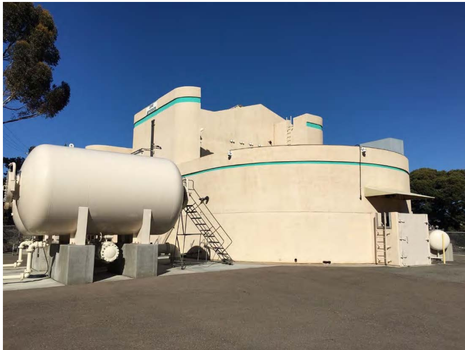
Buena Vista Pump Station
