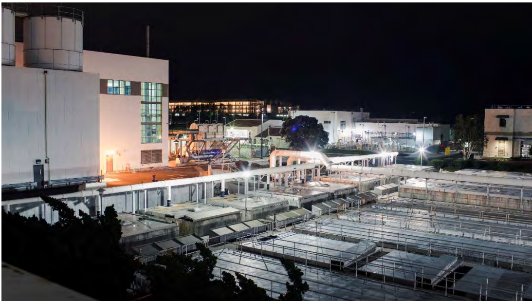
Primary Treatment Area
