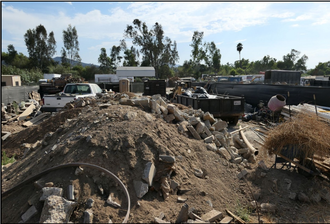
PHOTOGRAPH 2 Debris along Construction Option 2, Looking Southwest
