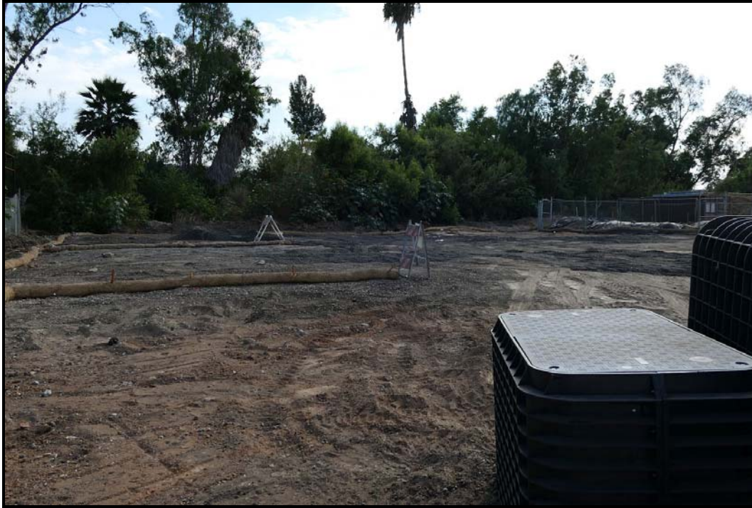
PHOTOGRAPH 3 Disturbed Soils in Construction Option 2, Looking Southwest
