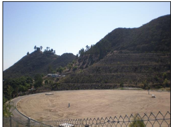
The Twin Oaks Reservoir site houses two buried reservoirs with a total storage volume of 73 MG adjacent to the SDCWA Twin Oaks Plant. The North Twin Oaks Reservoir is also shown on a hill in the background.
