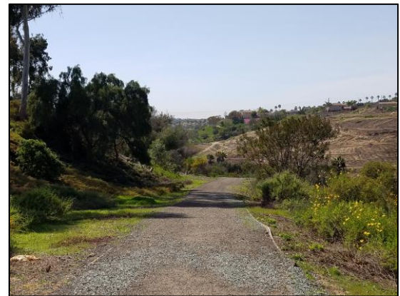
The Land Outfall is a critical component of the District's infrastructure. The alignment includes narrow easements along environmentally sensitive corridors and major streets.
