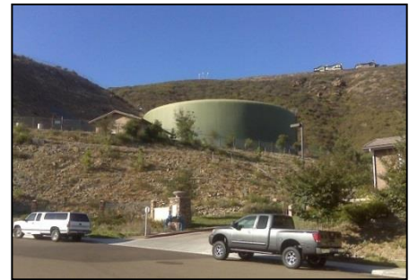
The 877 Reservoir and the 1115 Pump Station serve new development in San Elijo Hills. The reservoir helps regulate flows from VAL-7 in the 877 Zone.
