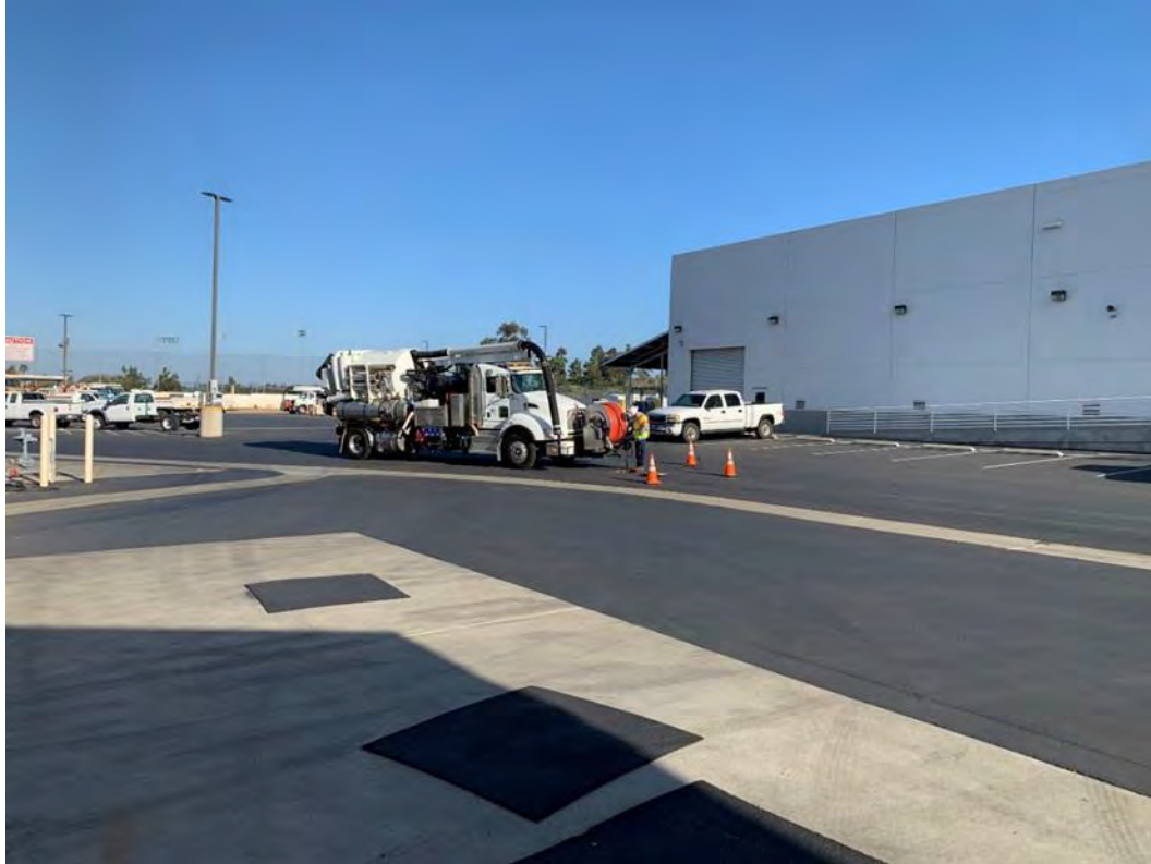
Figure 5: Combination Truck Response Team #2 at Downstream Manhole
