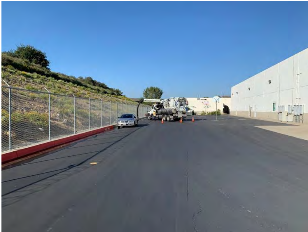
Figure 4: Combination Truck Response Team #1 at Downstream Curb & Gutter
