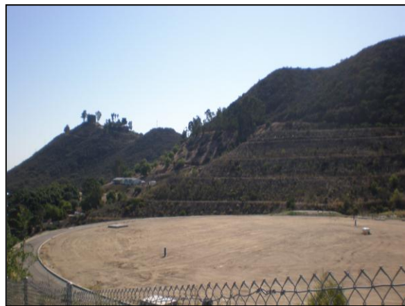
The Twin Oaks Reservoir site houses two buried reservoirs with a total storage volume of 73 MG adjacent to the SDCWA Twin Oaks Plant. The North Twin Oaks Reservoir is also shown on a hill in the background.
