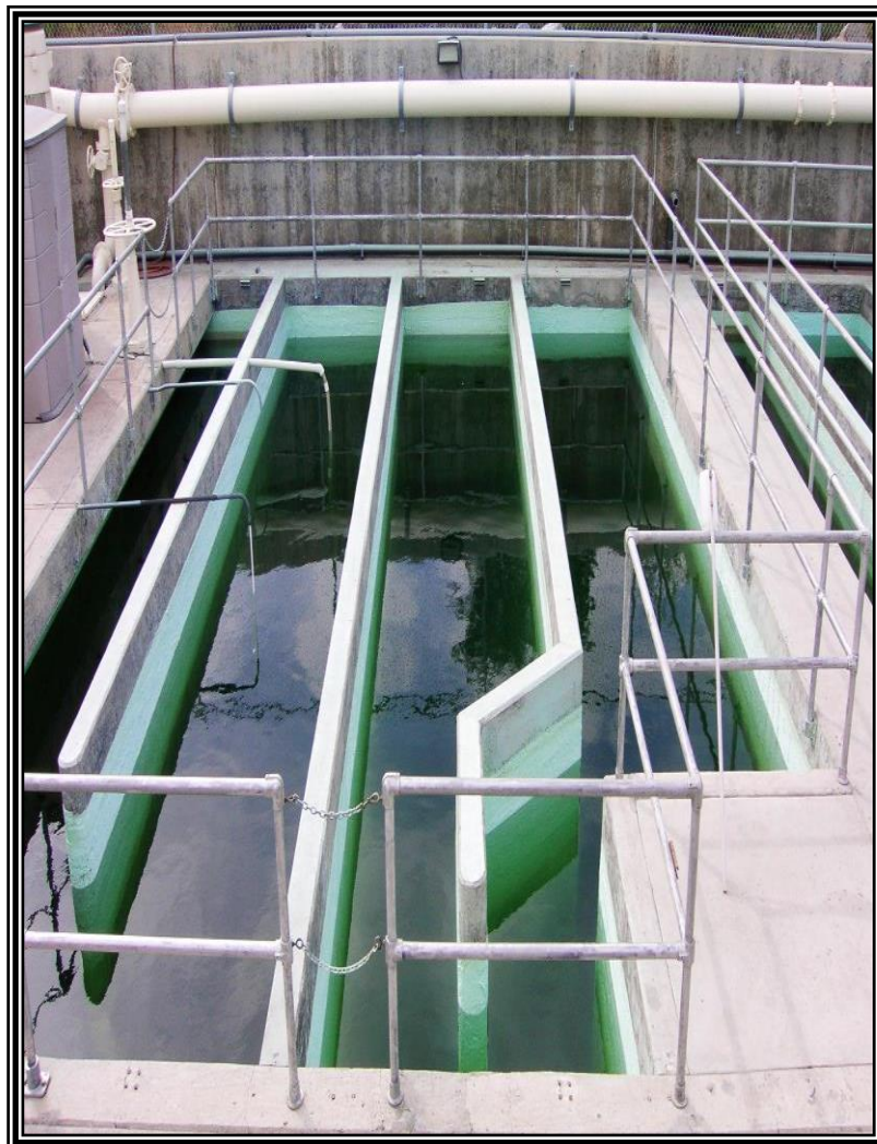
Chlorine Contact Tank at Meadowlark Wastewater Reclamation Facility
